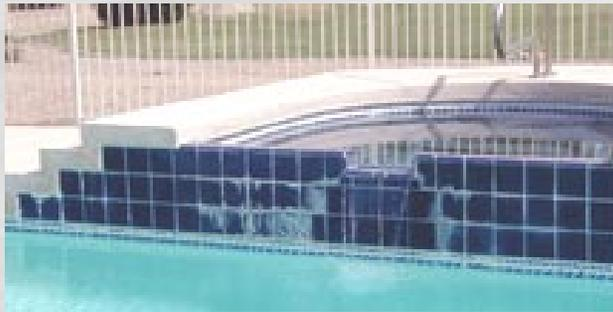
Fountain and pool tile cleaning with abrasive blasting is a safe and effective technique for removing calcium and scale deposits.
